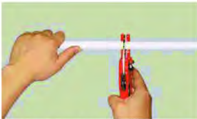
1. Cut pipe at right-angles using a pipe cutter.
