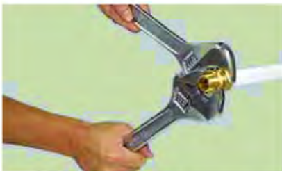
5. Use a spanner to tighten it up completely.
