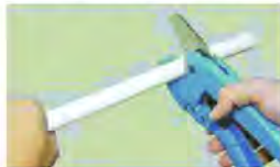
Step 1:Pipe Cutting
